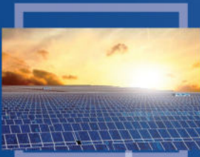
SOLAR TARLALAR SOLAR POWER PLANTS
