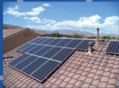
EV SİSTEMLERİ ÇATI MONTAJI ROOF STRUCTURE FOR HOME SOLUTIONS
